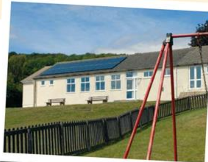
Newly-refurbished Randwick Village Hall with efficient double glazed windows and solar photovoltaic system on display
