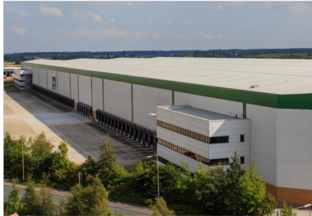
Up to 500 staff will work in the 550,000 sq ft warehouse in Sherburn-in-Elmet
