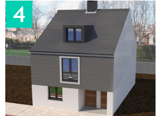
Step 4: Modular roof fitted
