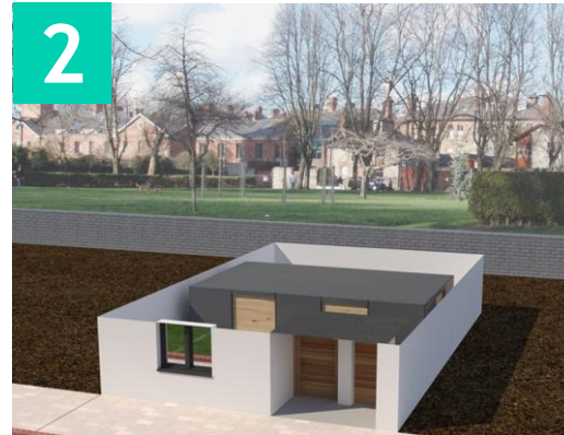
Step 2: External walls fitted
