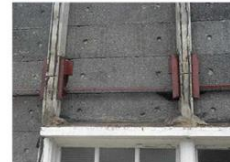
Bracing detail between columns
