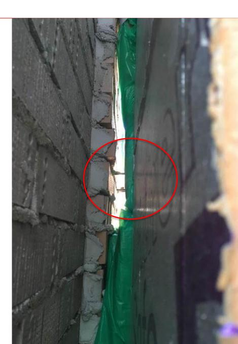
Make shift of three number lamatherm cavity Barriers butted together to make up the full cavity width
