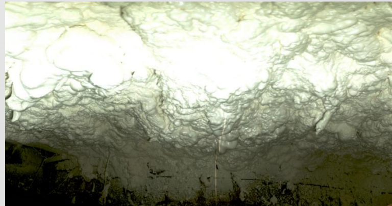
After the installation
