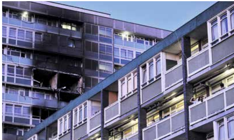
Fire safety failings were uncovered after a fire at Lakanal House, south London
