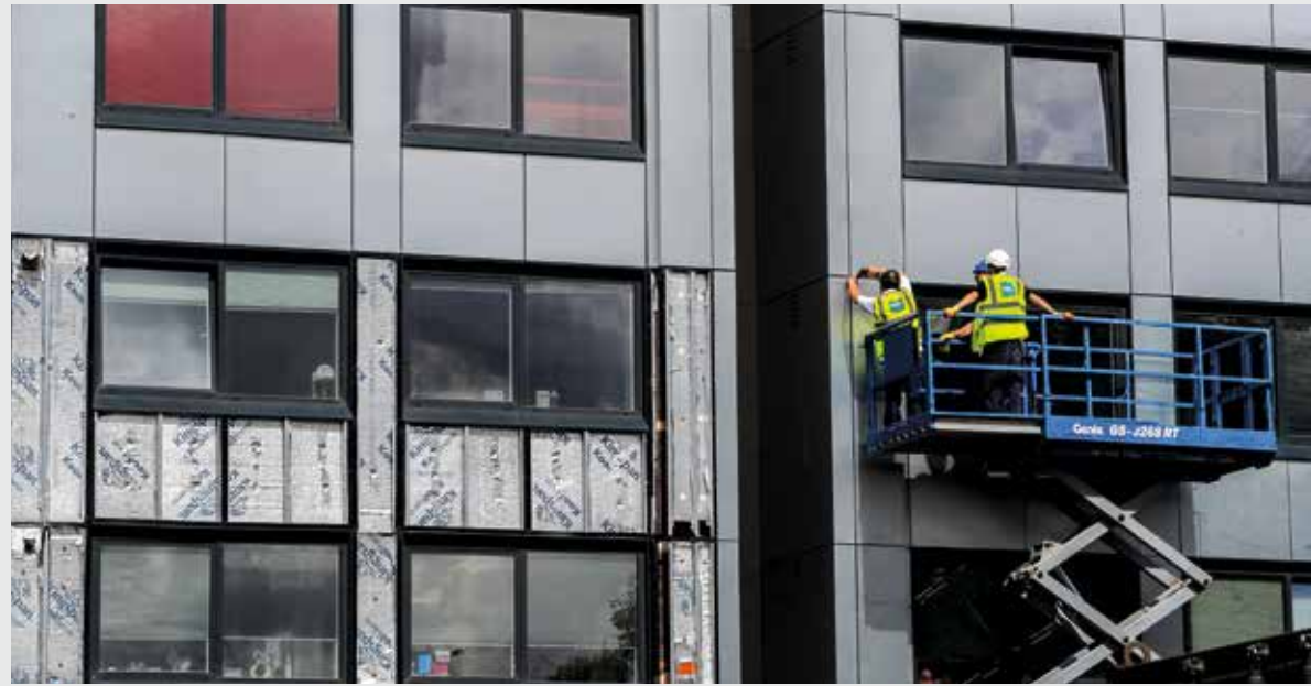
Cladding is removed from Whitebeam Court, in Pendleton, Greater Manchester, in the wake of the fatal fire at Grenfell
